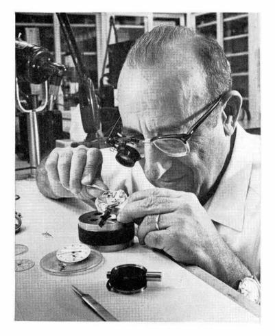
INSTALLING the balance wheel in a stop watch is a relatively easy task for Sol Azouz, a former watchmaker.
